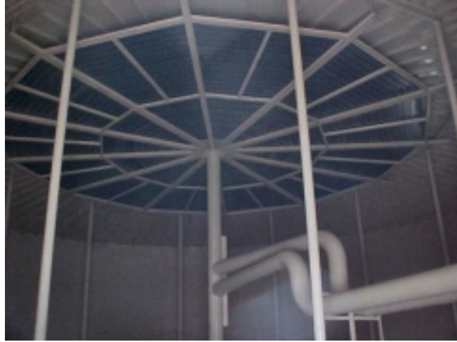
Photo E – Inside Thermal Energy Storage Tank
